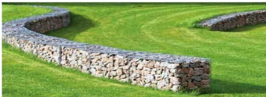
GABION BASKET RETAINING / SEAT WALL
