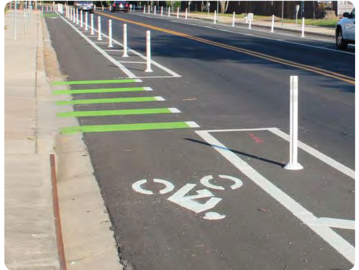
Figure 24 - Separated Bike Lane
