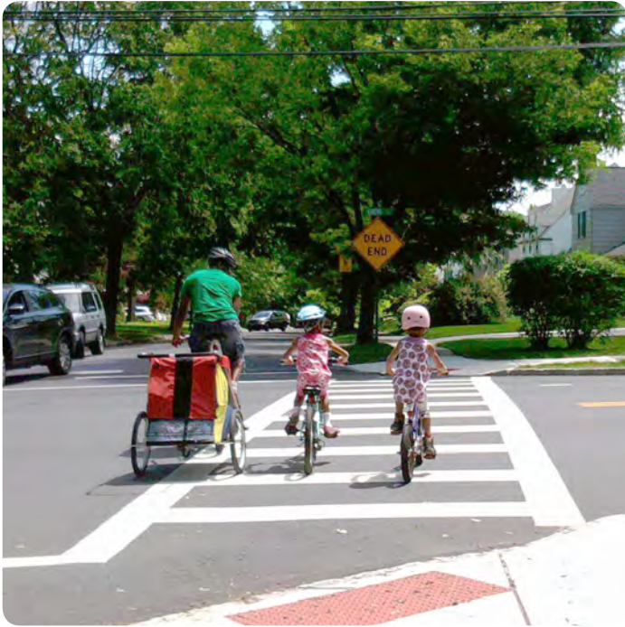
Figure 31 - High-Visibility Crossing Marking
