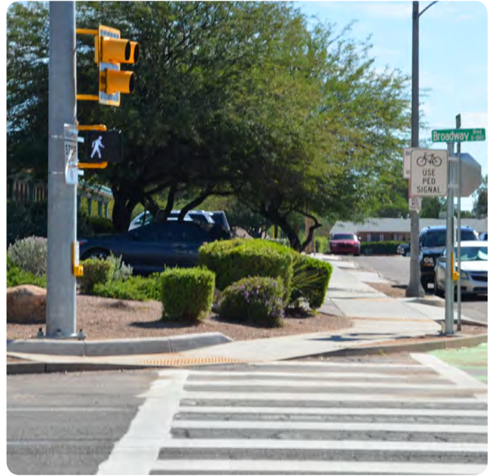
Figure 34 - Crossing Marking with On-Demand Signal
