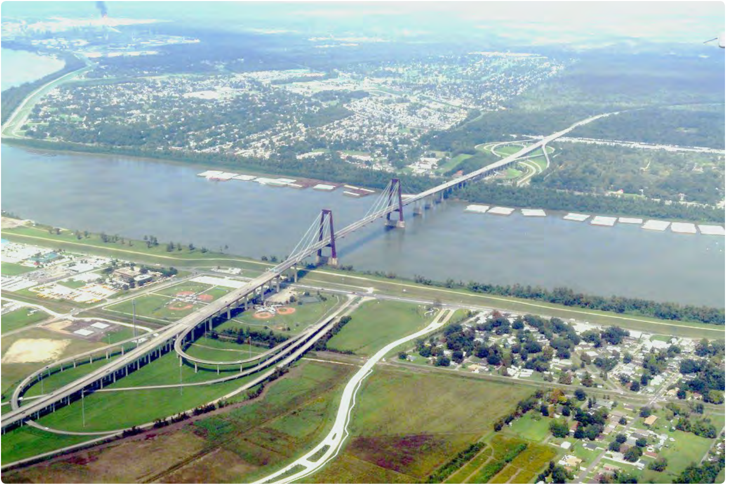
Figure 54 - Aerial View of Hale Boggs Memorial Bridge
