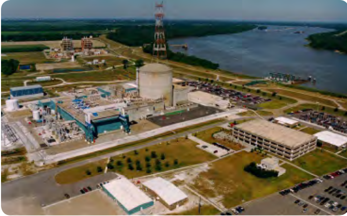
Figure 13 - Entergy's Waterford 3 Campus on the West Bank, facing Upriver
