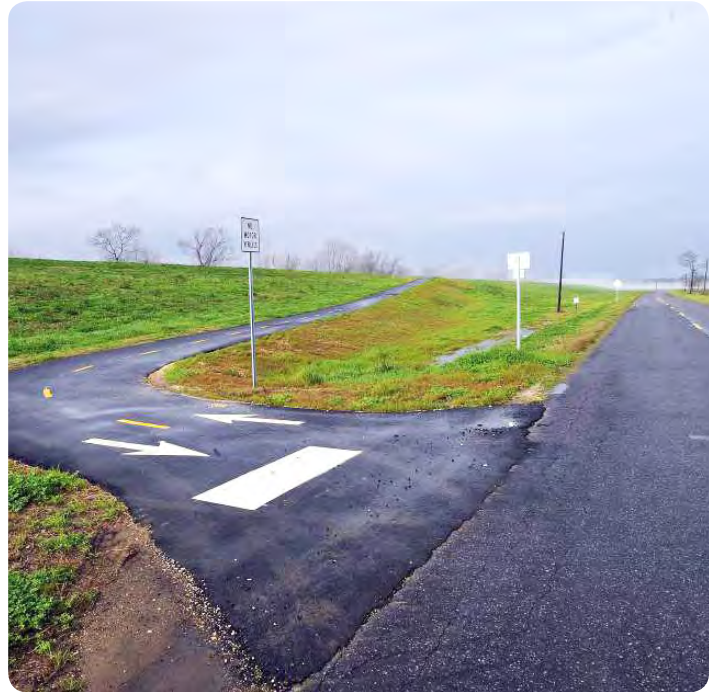
Figure 30 - Levee Access Path
